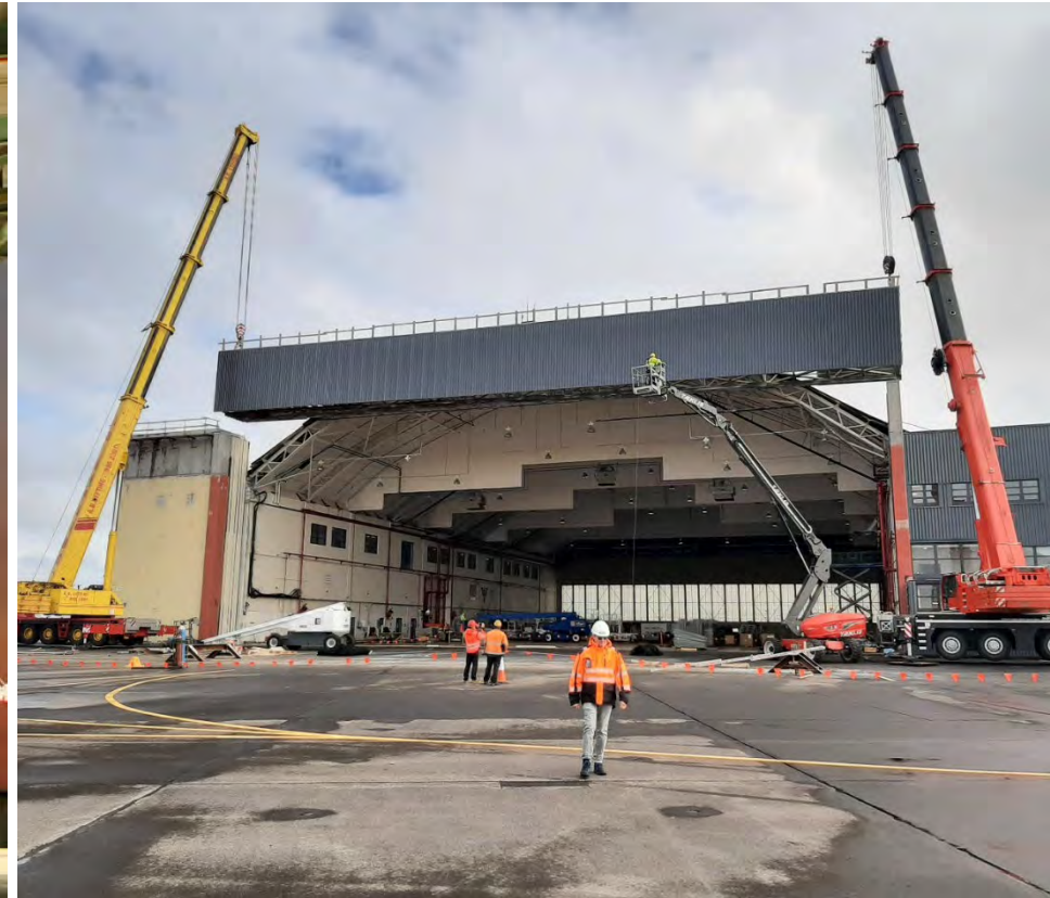
Hangar Renovation, Keflavik, Iceland
