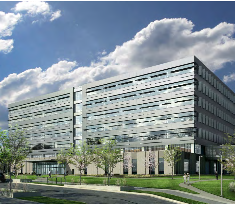
East Campus Building #4, Ft Meade, MD
