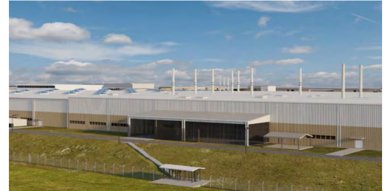
NAVFAC SE - Powertrain Phases II-VI NAS CORPUS CHRISTI, TX | Constr. Cost $350M+
