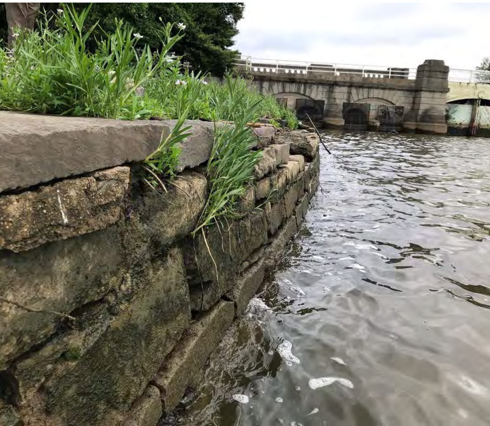
National Park Service Seawall Reconstruction, Washington, DC
