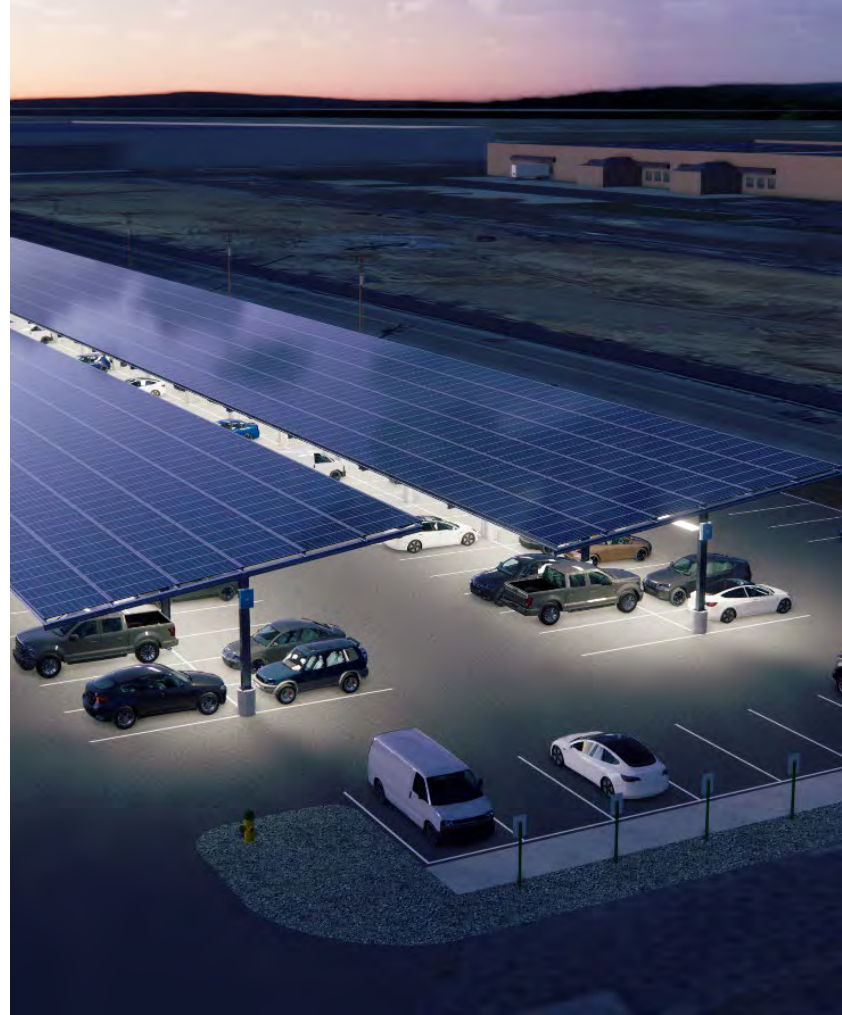
PV and Battery Storage, DLA Susquehanna, PA
