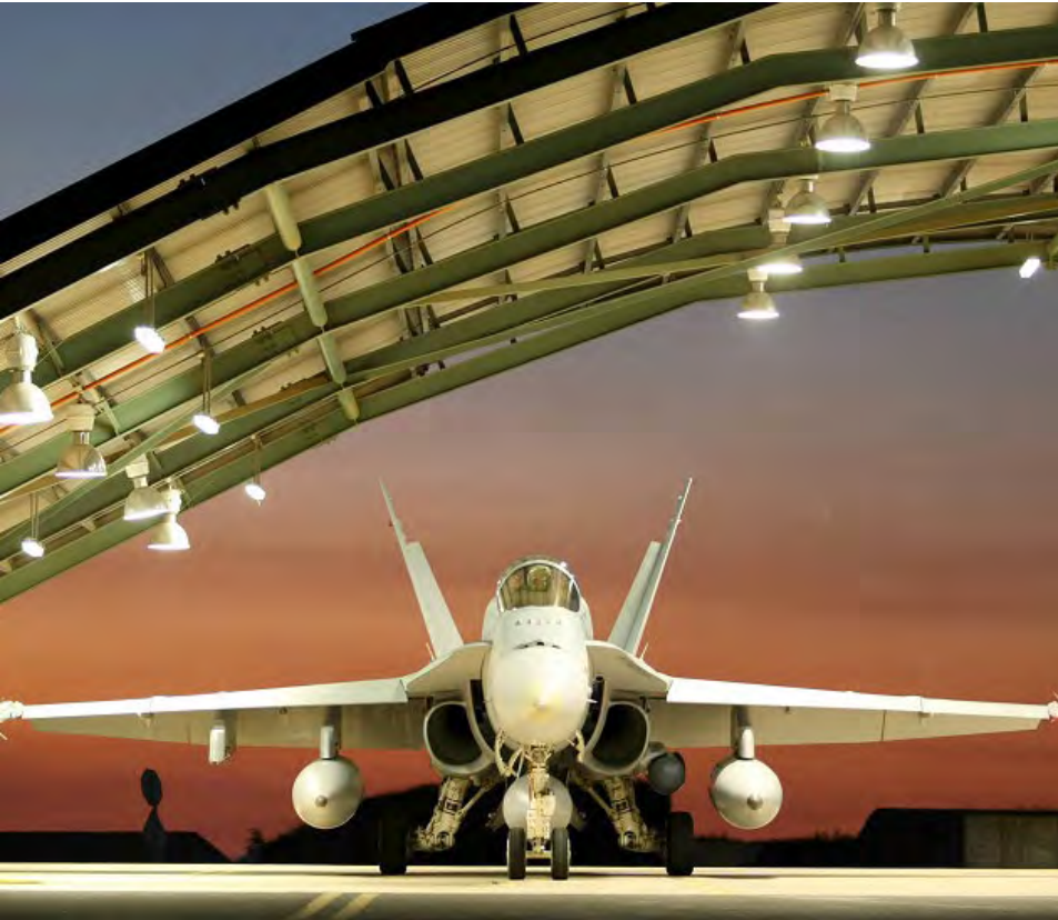
Riverina Redevelopment, Victoria and NSW, Australia
