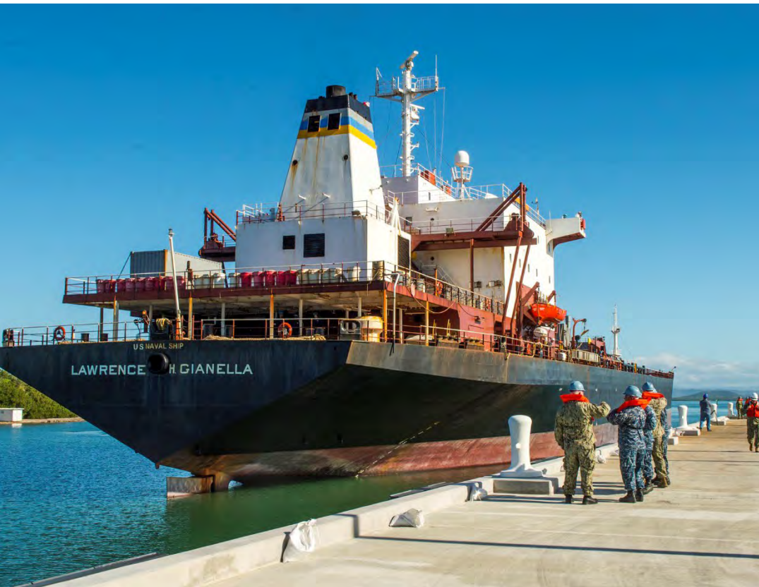
Pier Charlie Replacement, Naval Station Guantanamo Bay, Cuba
