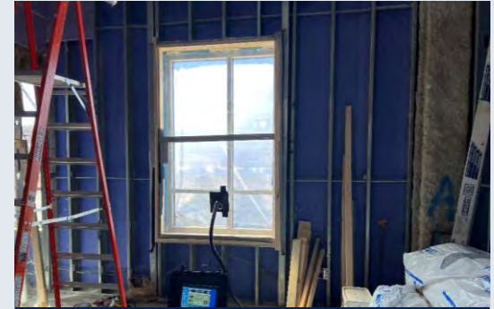
Window Leak Testing
