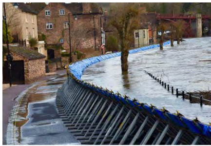
Modular Perimeter Flood Barrier
