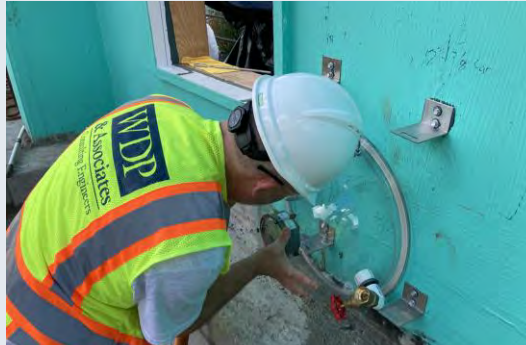
Air Leakage Testing
