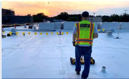
Roof Impedance Scanning
