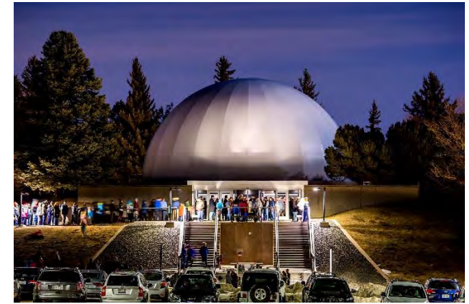
USAFA Planetarium Renovation USAFA, CO
