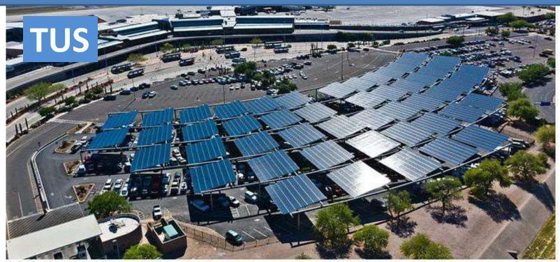
The Tucson International Airport has a uniquely designed "solar amphitheater" producing 1.25 MW. The project faces southeast to meet FAA anti-glare best practices. Barker Morrissey Contracting, Natural Power and Energy and Kyocera Solar assisted on the project, which used "Made in the USA" components. The airport plans on a 2.5-MW expansion sometime this year. (Credit: Natural Power and Energy)
