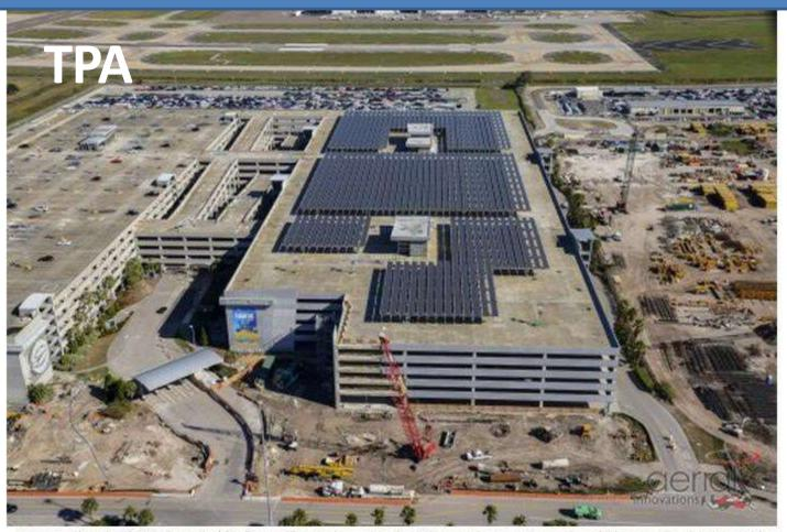
Tampa Electric (TECO) installed its first utility-scale system in 2015 at Tampa International Airport. The 2-MW parking canopy is on top of a parking garage. Florida's Solar Source installed the project, which is a one-of-a-kind concrete structure. (Credit: Solar Source)
