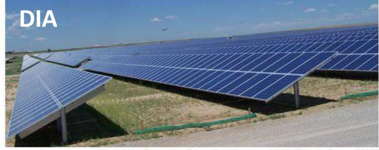
Denver International Airport has four solar farms (totaling over 10 MW), including a 4.4-MW project commissioned in 2011 and owned by Constellation. Some of the electricity produced is used directly at the airport, and the rest is sold back to the grid. The airport has a total of 42,358 solar panels spread across 55 acres of solar fields. (Credit: Constellation)
