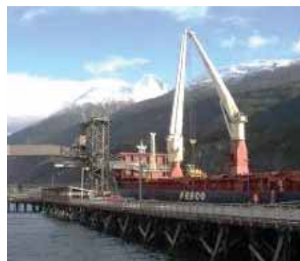
Skagway Ore Terminal and ship loader. Photo courtesy AIDEA
