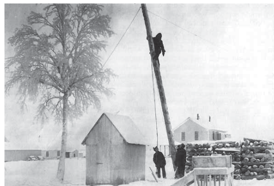
Telegraph repair at Fort Gibbon, Alaska. Photo courtesy U.S. Army Center of Military History
