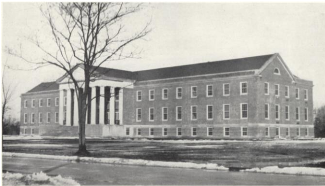
Post Headquarters Building, Fort Belvoir, Virginia
