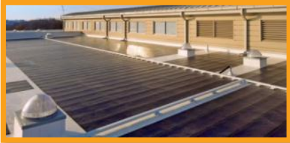
356kW Thin-Film PV Roof Systems
