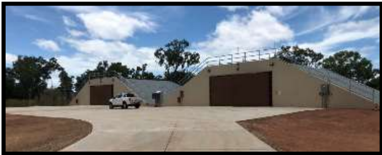
RAAF Tindal: Earth Covered Magazines
