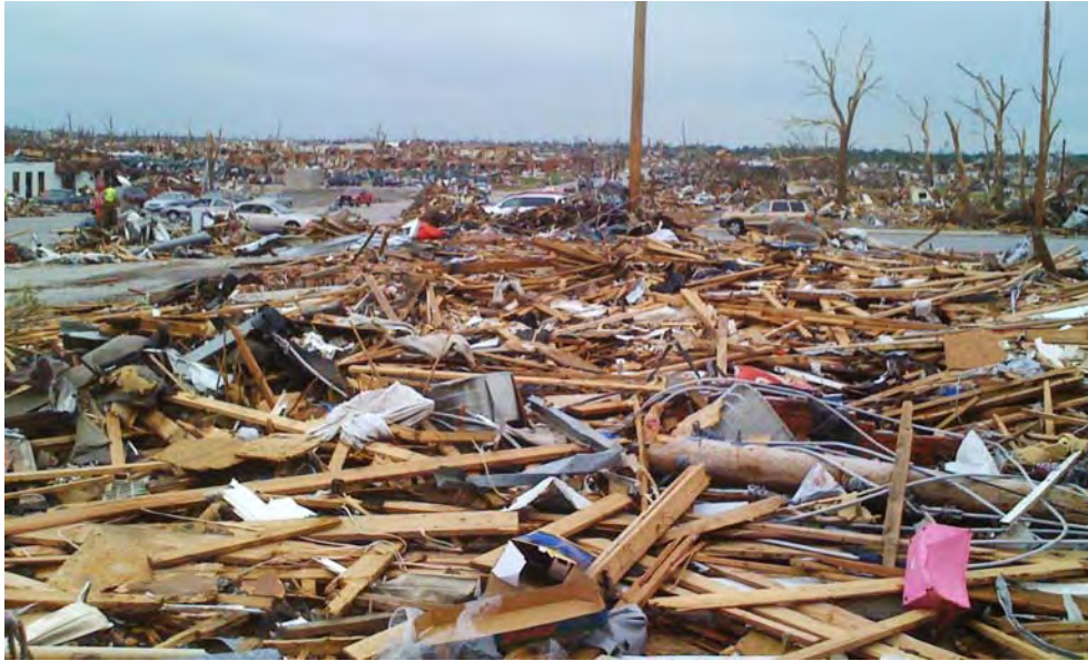
To lead collaborative efforts to identify and resolve national security infrastructure-related challenges. Photo Credit: Michael Goldschmidt, AIA – S.A.V.E. BECOME INVOLVED
