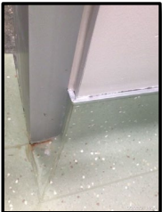
Repair drywall above base trim cap
