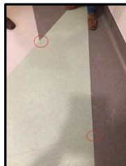
Repair pin holes in marked locations
