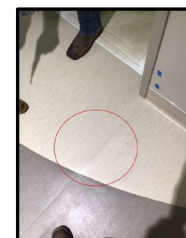
Floors is lifting at seam. Repair weld
