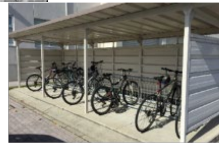
Metal shelter, high walls
