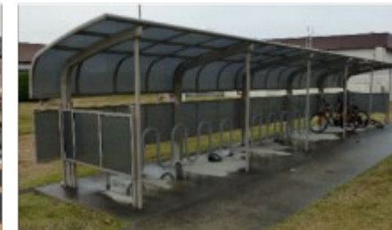
Fiberglass shelter, cantilever
