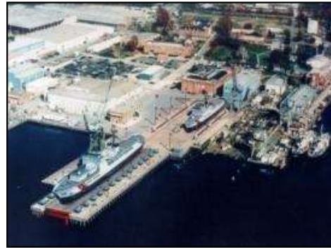
Industrial Facilities & Bases
