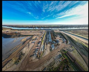
USACE Sacramento Weir Widening, \$173M: Granite is widening the weir and the constructing a new fish passage structure and a vehicular bridge connecting Old River Road to just north of West Sacramento.
