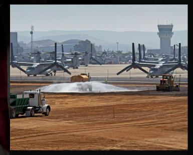
NAVFAC MV-22 LEED Gold Miramar Hangar Design-Build, \$107M: This design-build project consisted of a new hangar, tarmac parking apron/taxiway expansion, excavation, demolition, cement-treated base (CTB), white paving with on-site batch plant operations, and asphalt paving.
