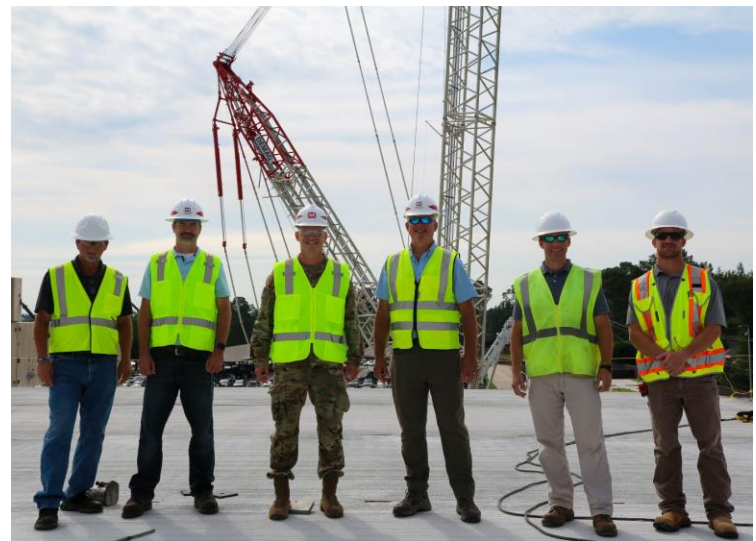
USACE personnel during the construction of a new parking garage at the Columbia Dorn VA Medical Center
