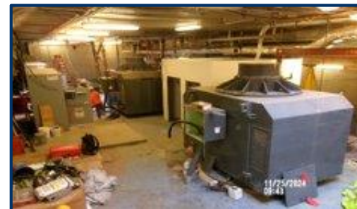
NNSY DD8 Pump Well Motor Install
