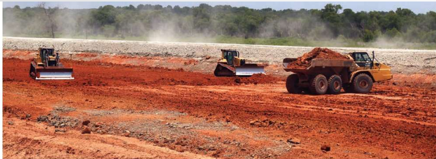
Contractors for the U.S. Army Corps of Engineers Tulsa District use heavy equipment to move tons of dirt while working on phase II of the Cumberland Levee Repair project along the Washita River, 12 miles east of Madill, Oklahoma. The levee was over-topped and breached June 21, 2015, during a record flood event brought on by historic amounts of rainfall across Oklahoma.
