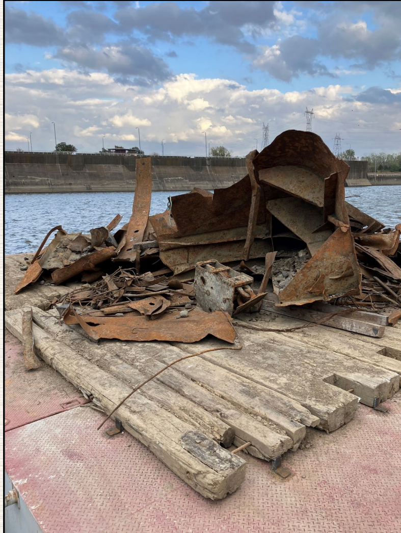
Existing Debris Removed from Scour
