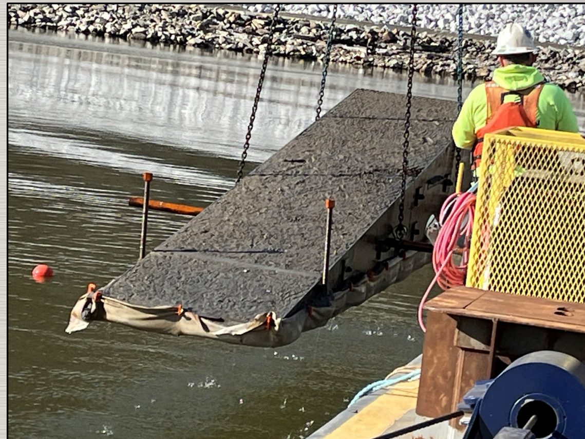
New Lift 2 Custom Sloped Formwork, Transition from Wall
