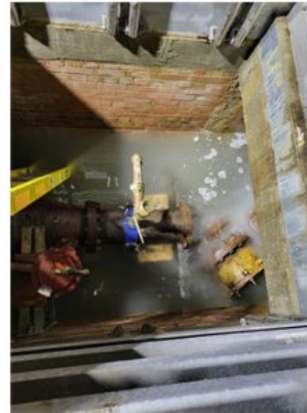
Water intrusion and repair photos at meter within vault
