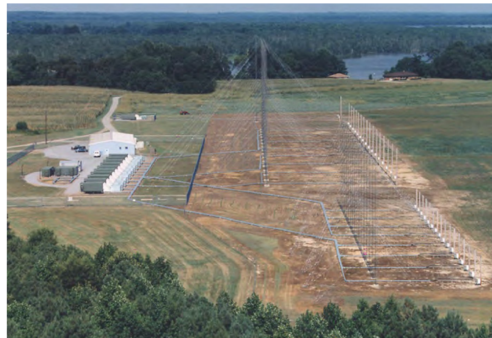
Example Transmit Site
