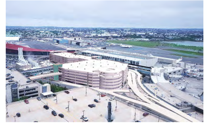
Terminal E Garage
