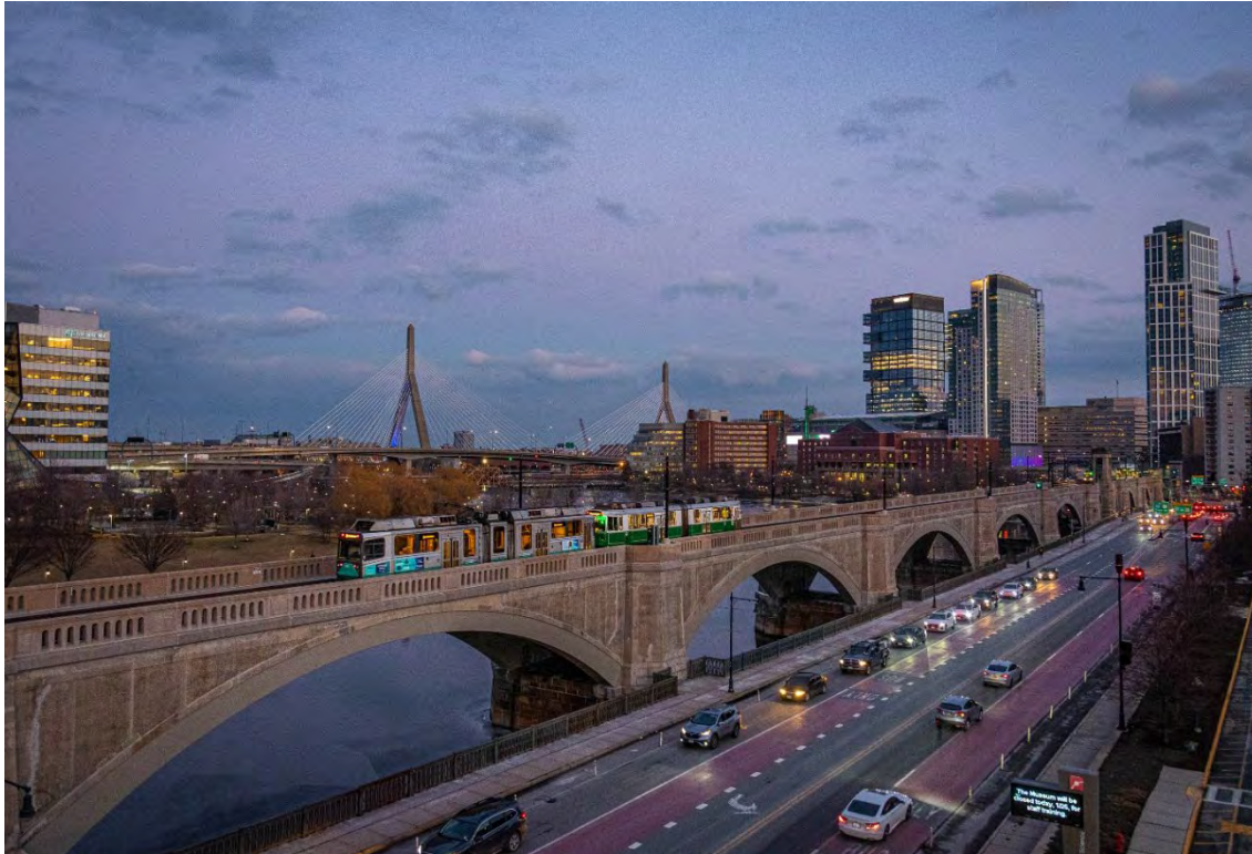
Green Line train passes over Lechmere Viaduct
