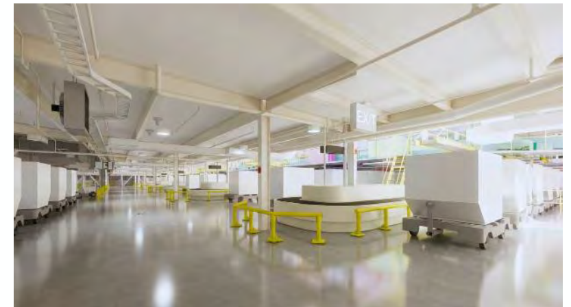
Terminal E New West Bag Room
