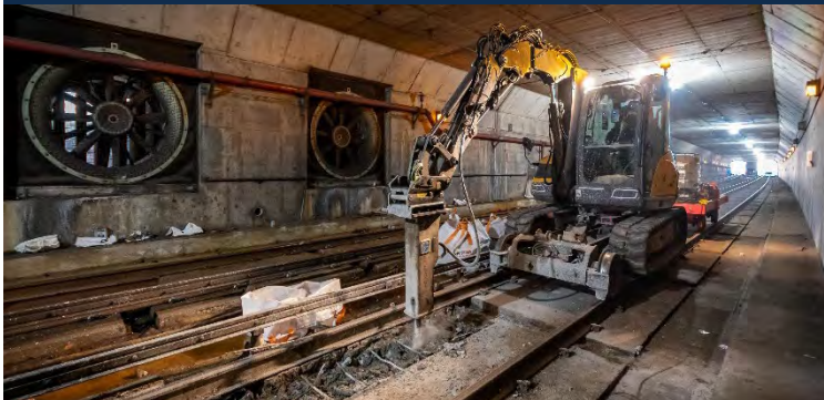
Maintenance work on the Orange Line Southwest Corridor
