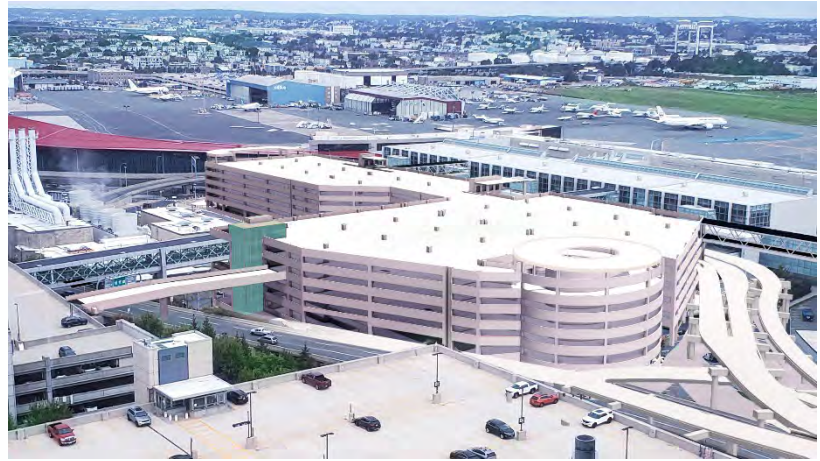
Construction of a 6-story, 2,100 parking space parking garage, connected with elevated pedestrian walkways to Terminal E and Terminal C and with a vehicular bridge to the adjacent West Garage
