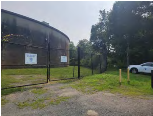
Existing MWRA Bear Hill Storage Tank, Stoneham (6MG)
