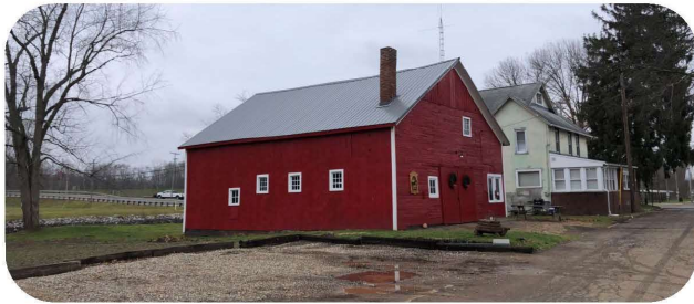
USACE Magnolia Levee Dam | Historic Structures Survey
