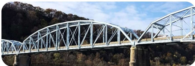
New Kensington Bridge Preservation | Bridge Inspection
