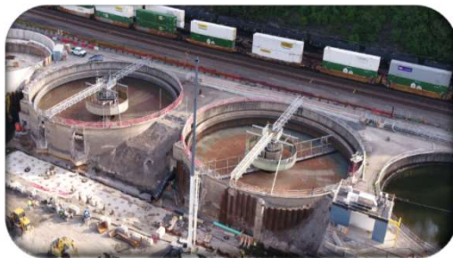
ALCOSAN Wet Water Plant Expansion | QA Inspections, Subconsultant
