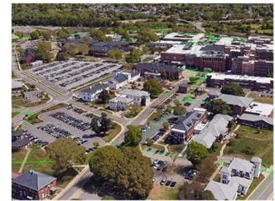
Hampton VAMC Sewer Rehab | Civil - Prime
