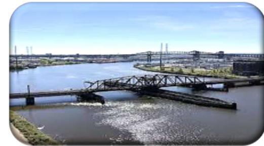
Consolidated Rail Corporation Point No Point Bridge Replacement | QA Inspections, Subconsultant
