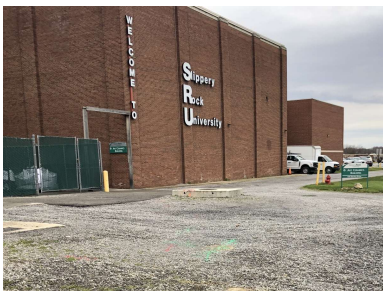
DGS – Slippery Rock Electrical Upgrade Civil, Survey - Sub
