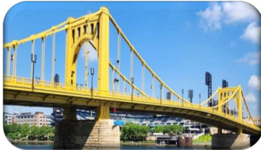
Pennsylvania Department of Transportation Roberto Clemente Bridge Rehabilitation | QA Inspections, Prime
