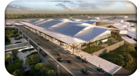
Allegheny County Airport Authority PIT Terminal Modernization Program | QA Inspections, Subconsultant
