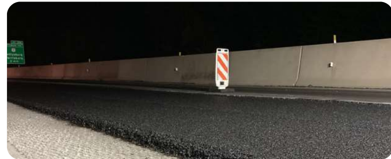
Pennsylvania Turnpike MP 235 Construction Inspection
