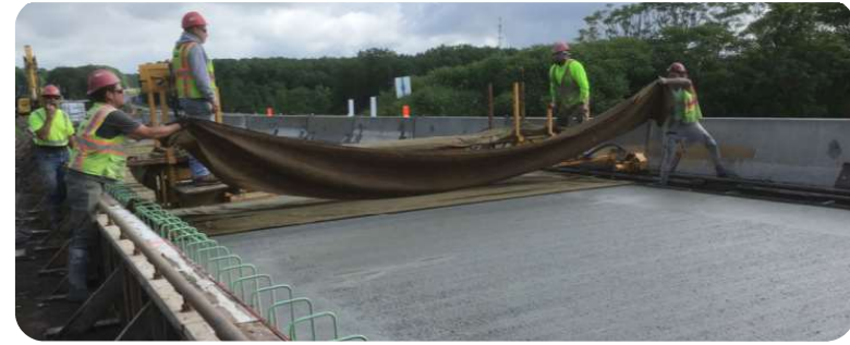
SR 79-A28 Crawford / Erie Counties Construction Inspection
