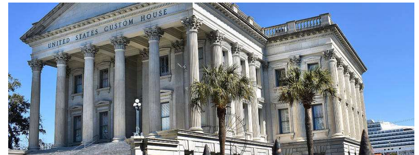
Chiller Replacement | Prime Contractor
