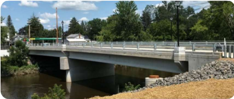
SR 006 Cambridge Springs Truss Construction Inspection
