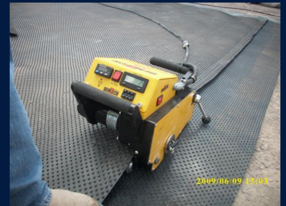
Double fusion welding
