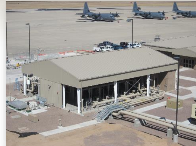
Cannon AFB – Fueling Facility
