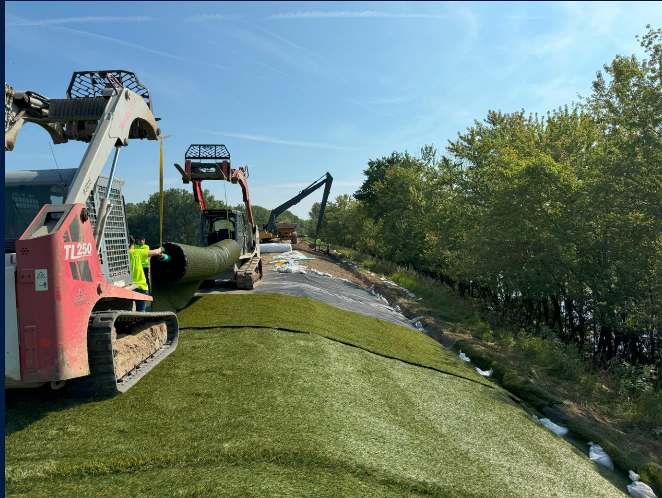
Turf Installation & Riverside Anchor Trench Installation
