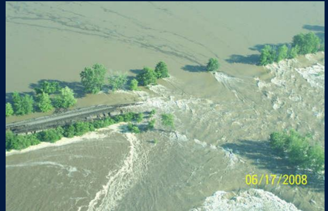
Gulfport, IL levee breach during the 2008 Mississippi River flood (Source: Quill Newspaper, 2008)
