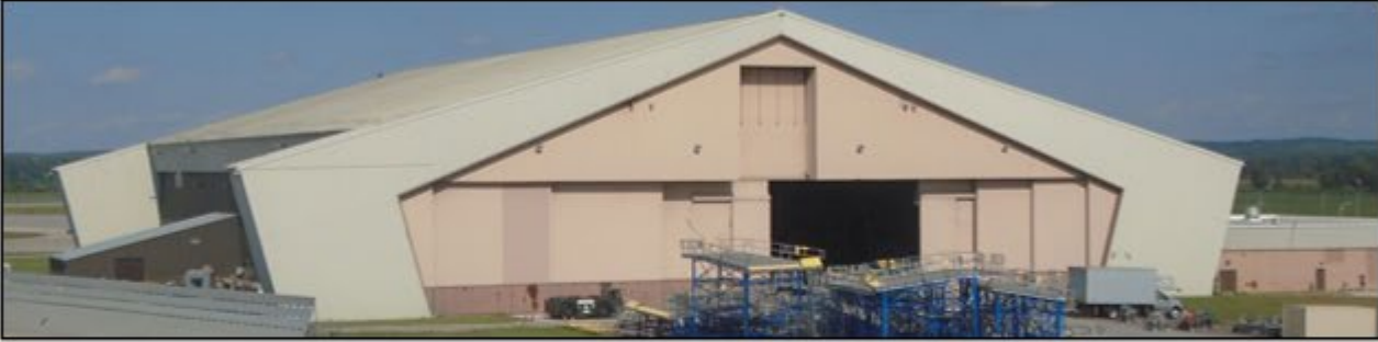
E4-B hangar 565 Repairs
