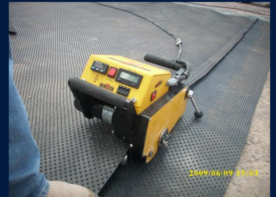
Double fusion welding
