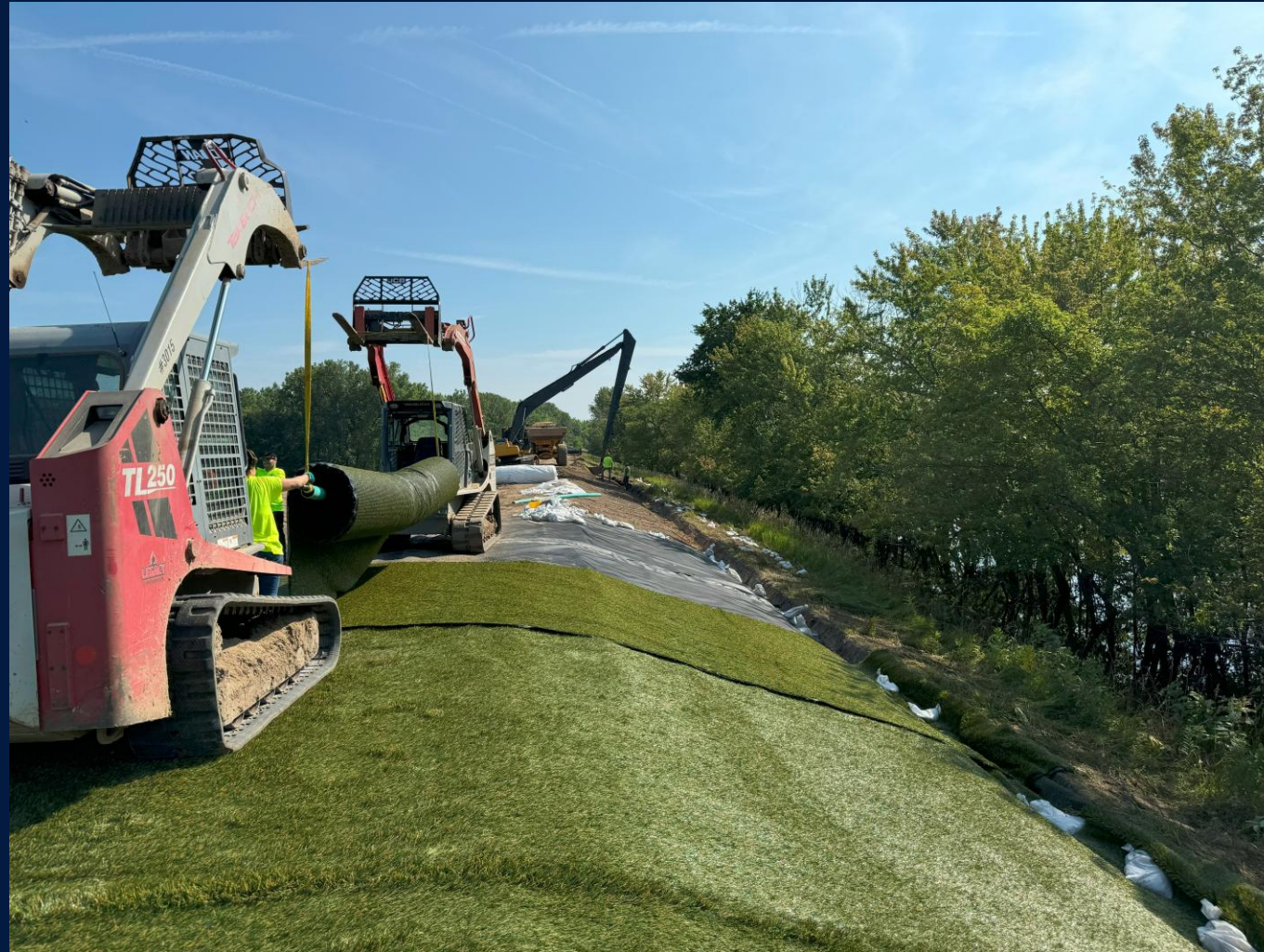
Turf Installation & Riverside Anchor Trench Installation
