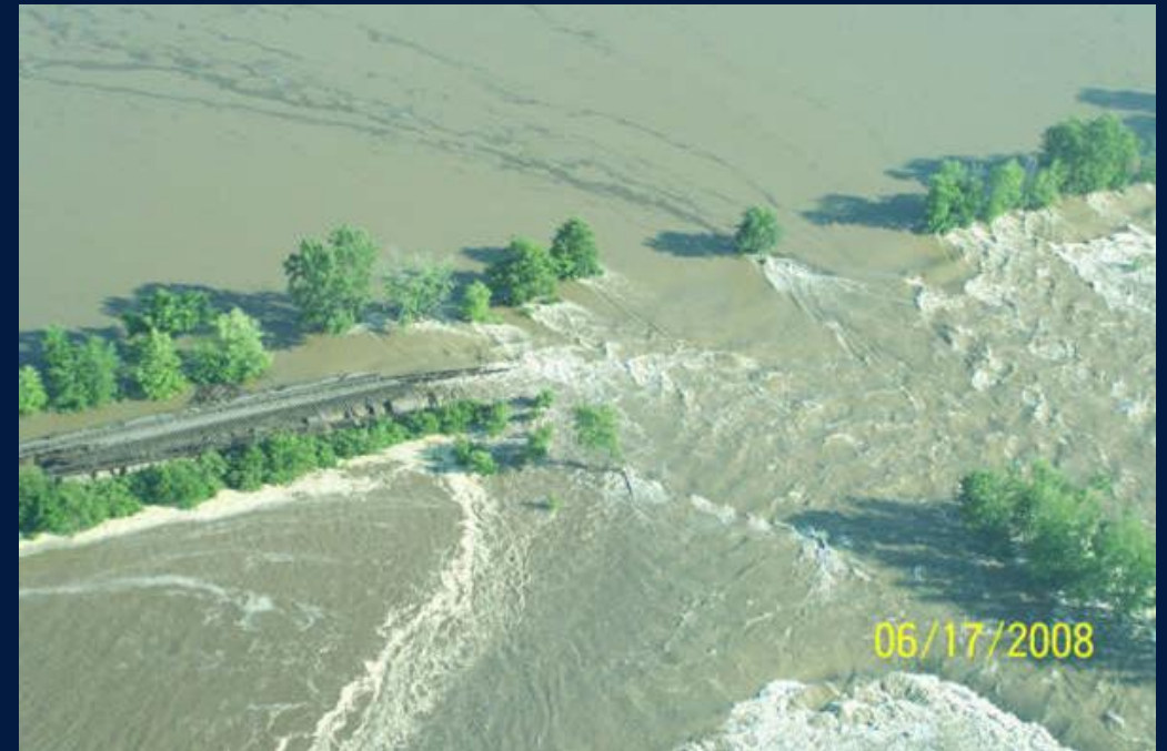
Gulfport, IL levee breach during the 2008 Mississippi River flood (Source: Quill Newspaper, 2008)
