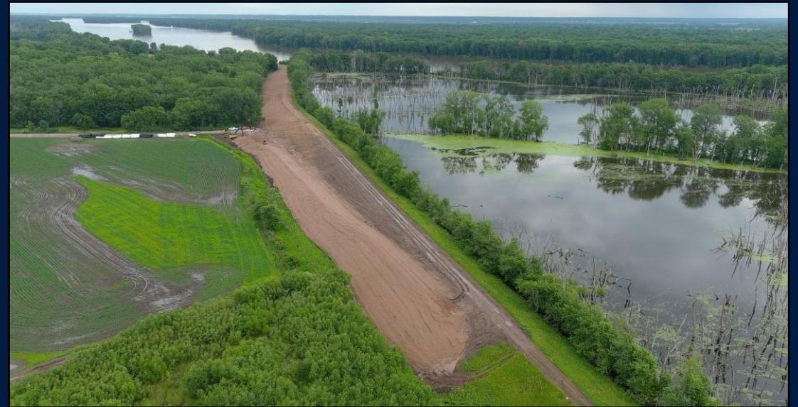
Rough Grading of the Muscatine Island Levee prior to HydroTurf Installation, June 2024.
