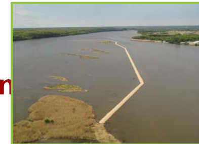
Starved Rock Breakwater
