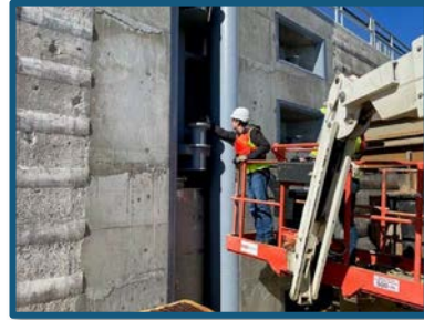
Lock 25 Phase 1 – Construction Complete
