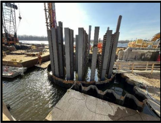
End Cell H-Piles being installed
