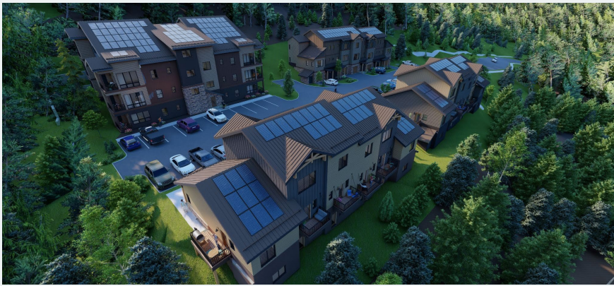
The Mountain Village, a completed modular project in Colorado. Courtesy of Shaw Construction
