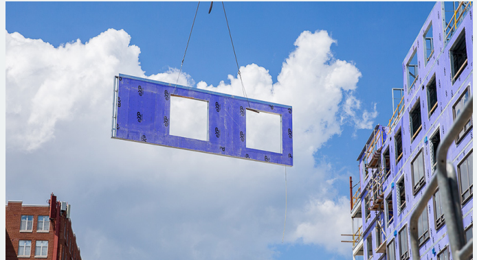
Panelized Wall. Courtesy of National Gypsum Company
