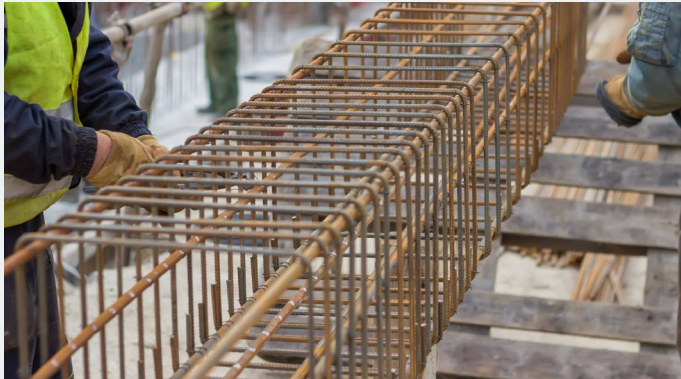
Prefabricated Rebar Cage. Image Courtesy of Hickman & Love
